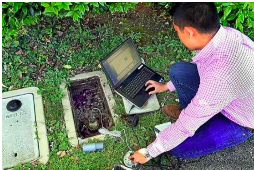
Energy Services installs a cellular water meter during the drought. Courtesy: Santa Cruz Sentinel.
