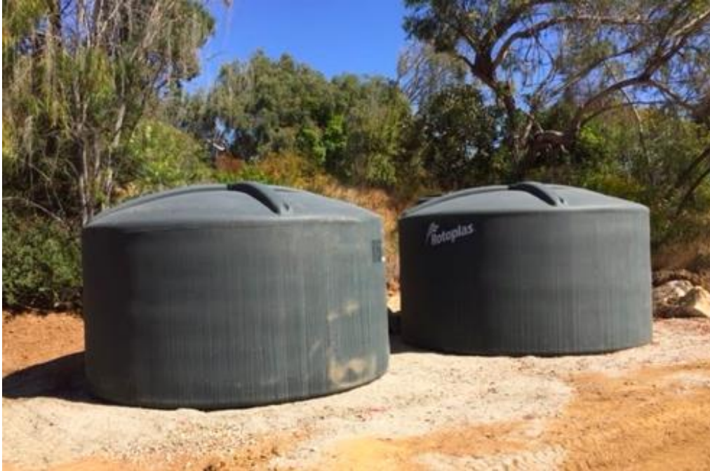
Two newly installed 6,000 gallon rainwater catchment tanks. Courtesy: Martin Quigley.
